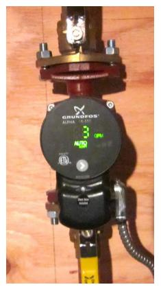
based on the circulator's power input, its RPM, and the internal calculation algorithms. They are capable of +/-5% accuracy when operated under the following conditions:
